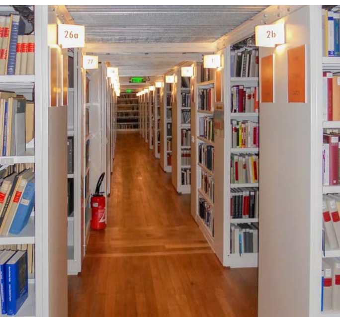
Load-spreading plinths were used to fit the double-level TwinSpace shelves onto the restored wooden floors.
