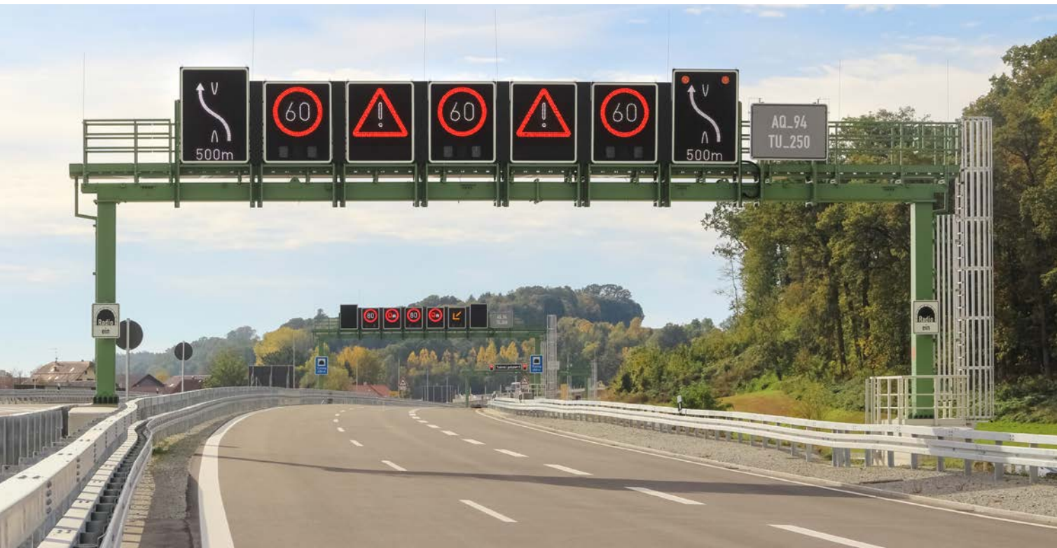
Altogether 15 gantries make sure that the traffic flows smoothly.
