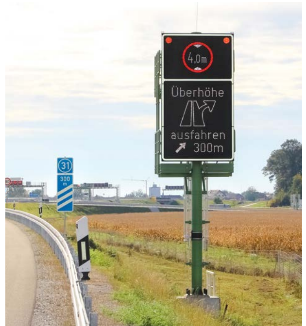
LED displays promptly send a diversion signal to excessively tall vehicles.
